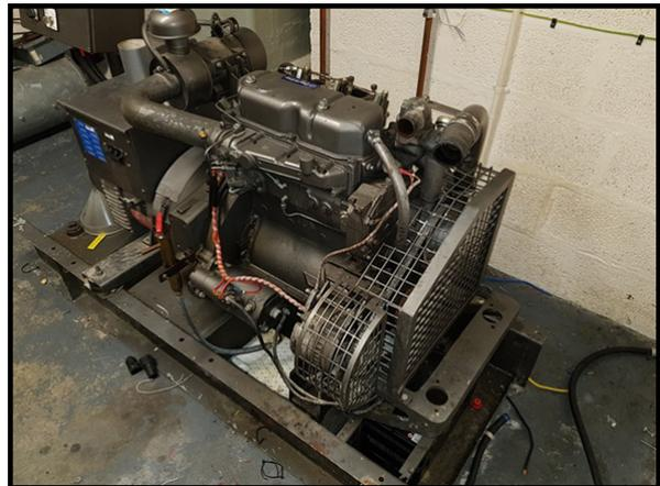
Newage/Stamford Type PC164E generator with Perkins Diesel Engine 3.152 series, 17.6kW, Serial Number: L7785/16 TO B.S. 5000/99, 380/415v (3 phase), 21.2 KVA, manufactured approx. 1987 with approximately 80 working hours.
