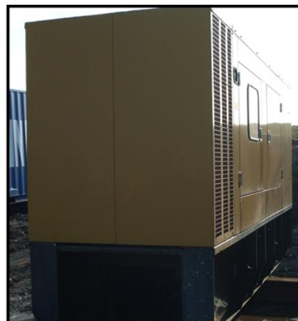
Olympian GEH275-4 generator, 200kW, 400 v (3 phase), 275 KVA, manufactured 2012 with approximately 9068 working hours.
