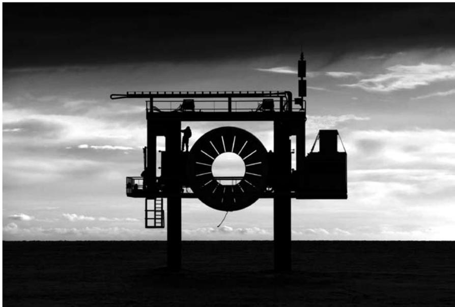
EMEC Tidal Turbine test rig at Falls of Warness, near Eday - Photo: Open Hydro, Mike Roper
