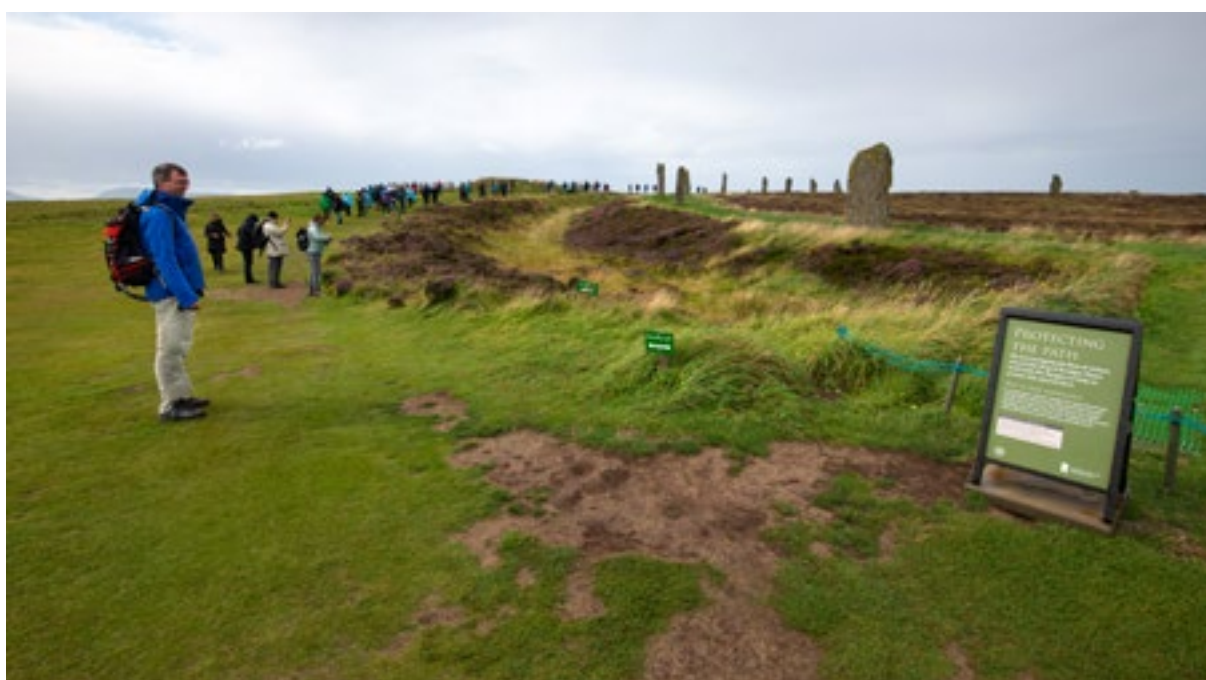
Visible signs of erosion at the Ring of Brodgar and the interpretation panel explaining to visitors why access to the interior of the site is prevented to protect it against erosion.
